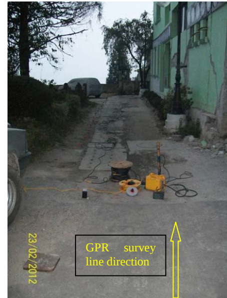
Fig. 9 GPR and MASW survey close to secretariat building
